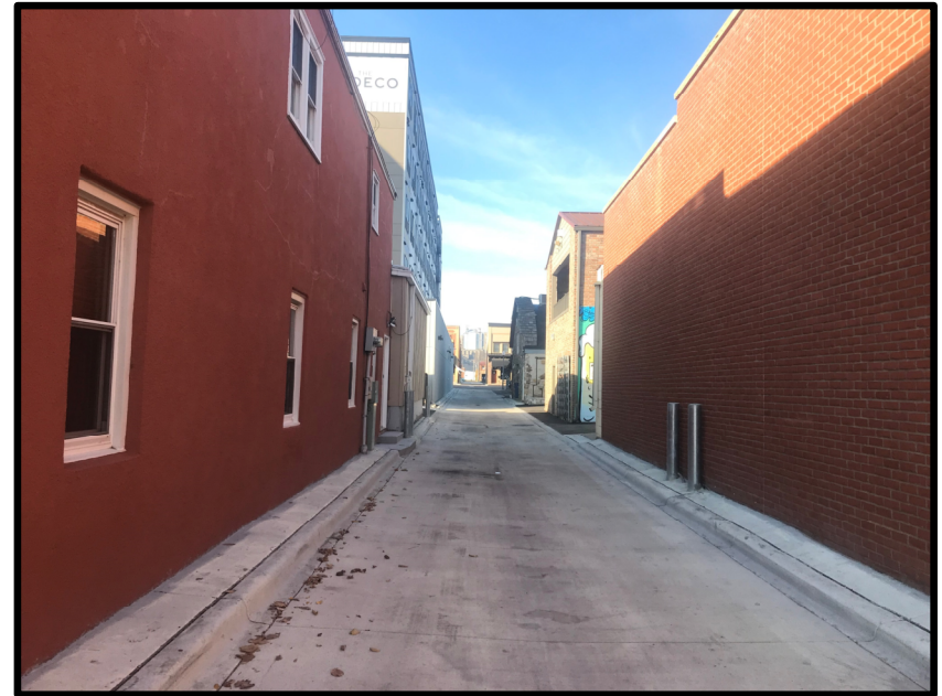
East Alley After Construction
