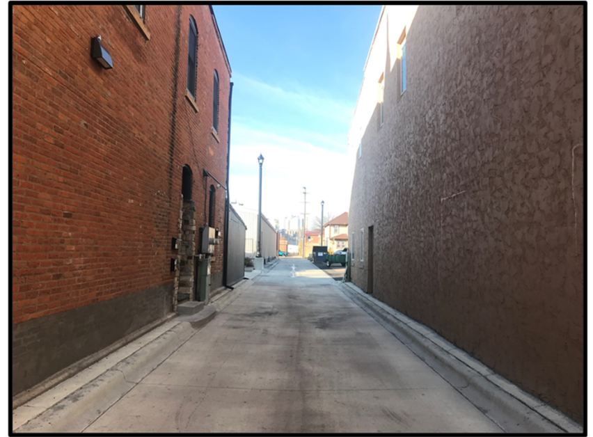
West Alley After Construction
