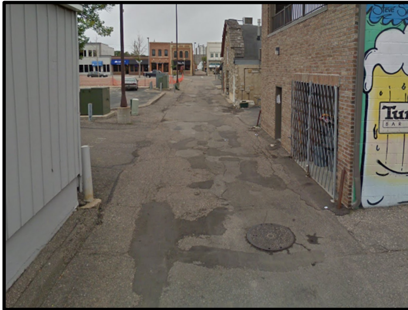
East Alley Before Construction
