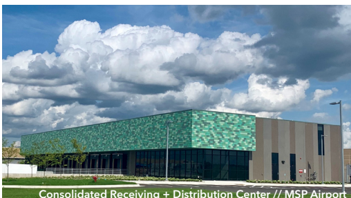
Consolidated Receiving + Distribution Center // MSP Airport
