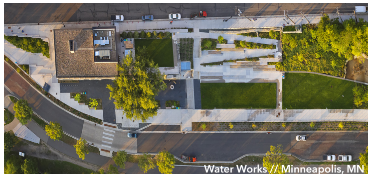
Water Works // Minneapolis, MN
