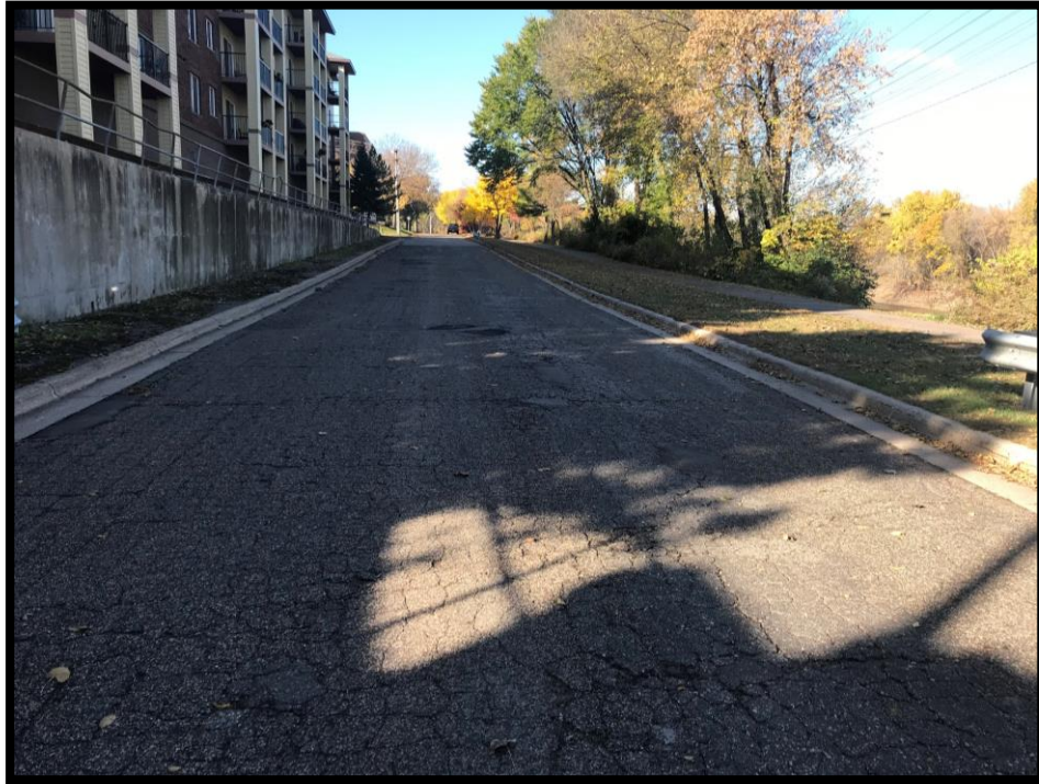
Levee Drive Before Construction
