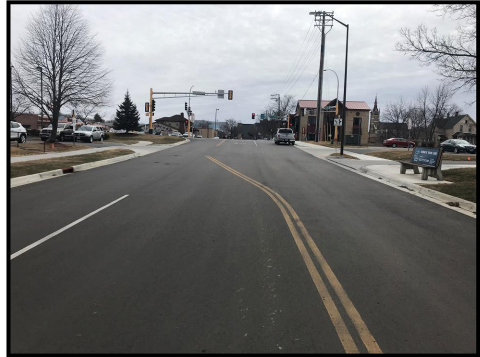
Fuller Street After Reconstruction
