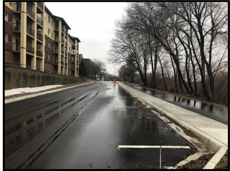
Levee Drive After Reconstruction
