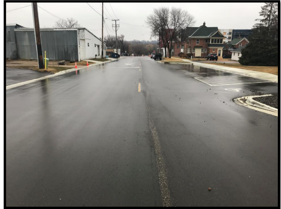
Scott Street After Reconstruction
