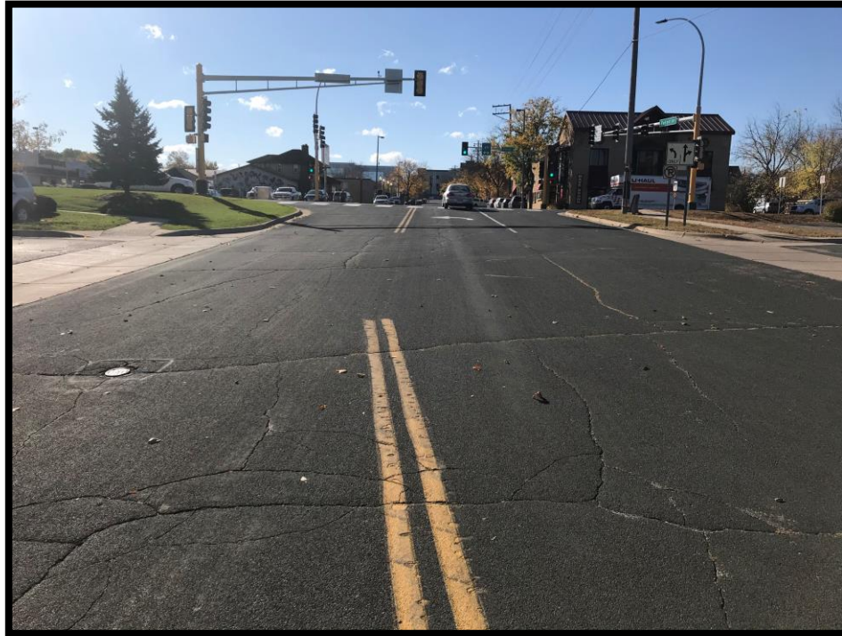
Fuller Street Before Construction
