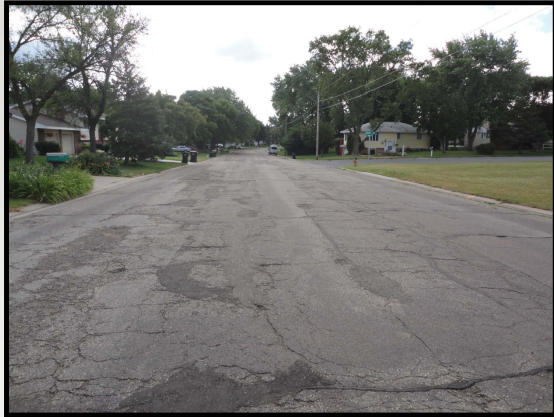
Shakopee Avenue – Before Construction
