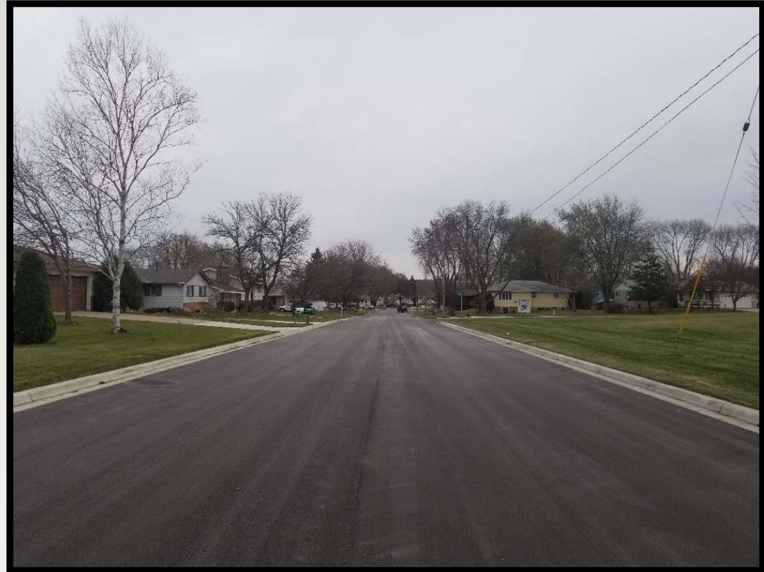
Shakopee Avenue – After Construction
