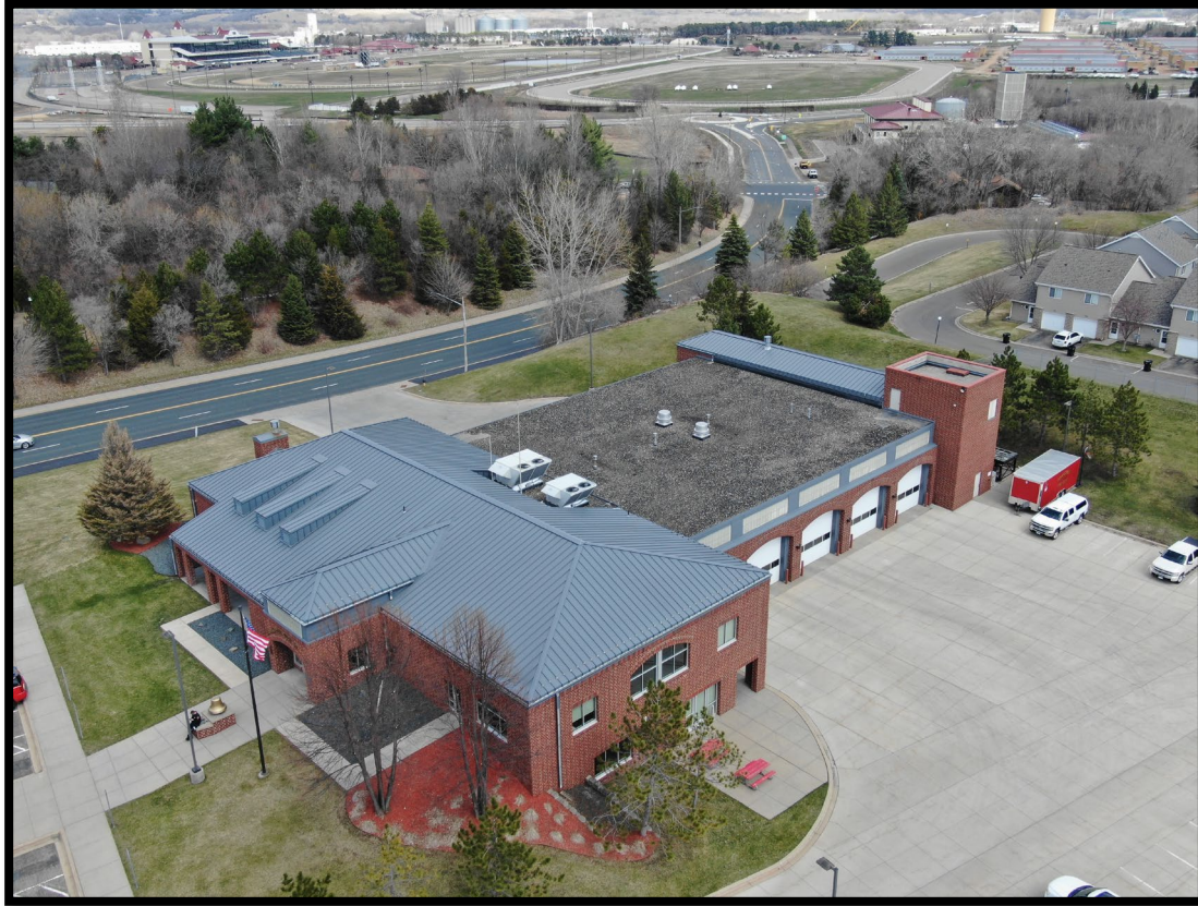
Fire Station One - 2700 Vierling Drive East
