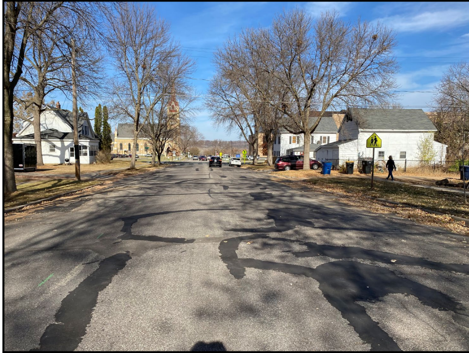
Atwood Street Before Construction
