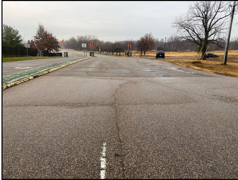
Valley Fair Drive Before Construction
