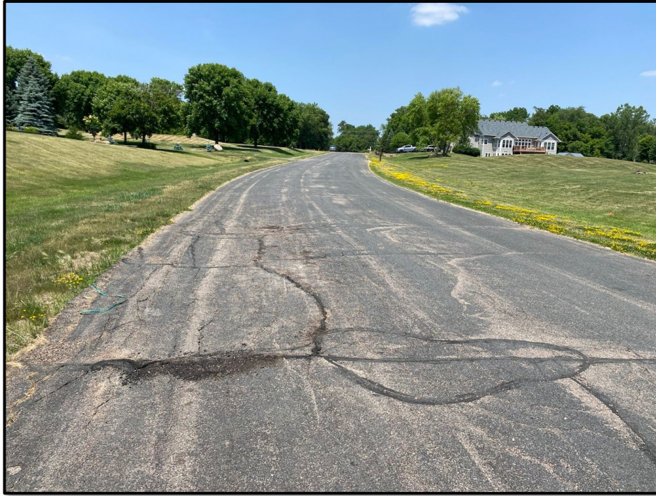
Dominion Hills/Maple Trail Estates Before Construction
