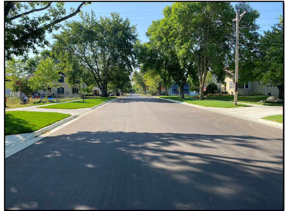
Atwood Street After Reconstruction
