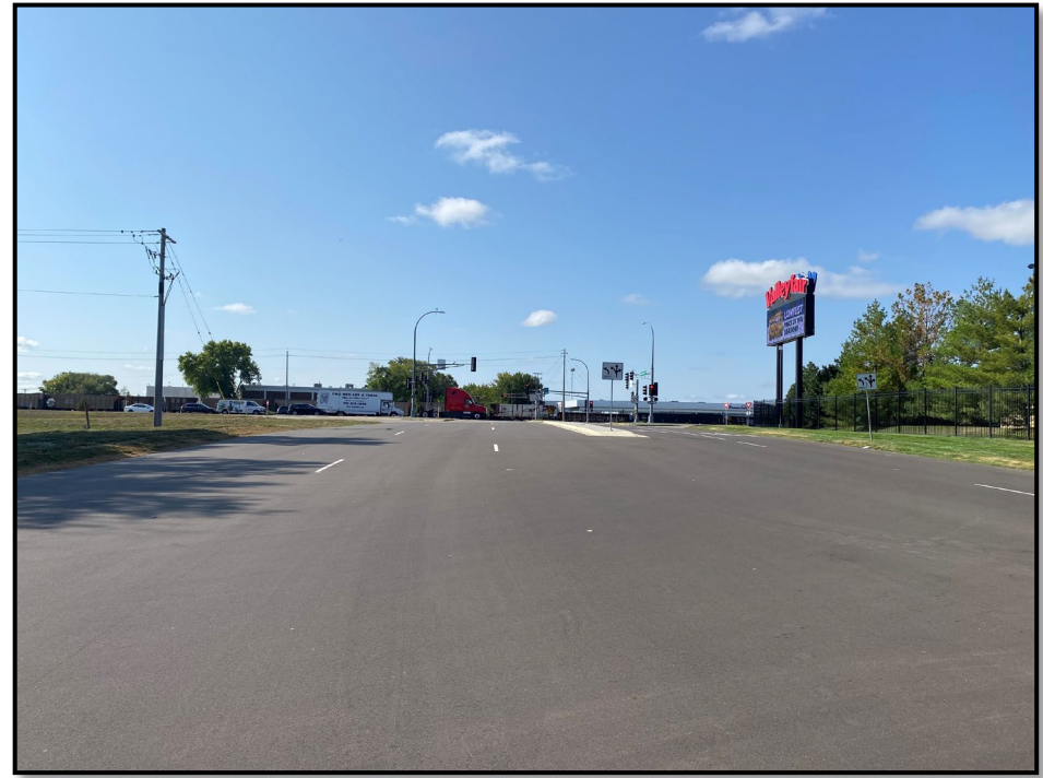
Valley Fair Drive After Reconstruction
