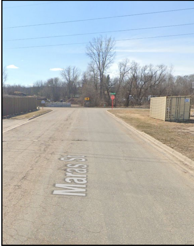
Maras Street Before Construction
