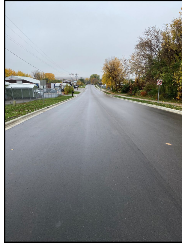
Maras Street After Reconstruction
