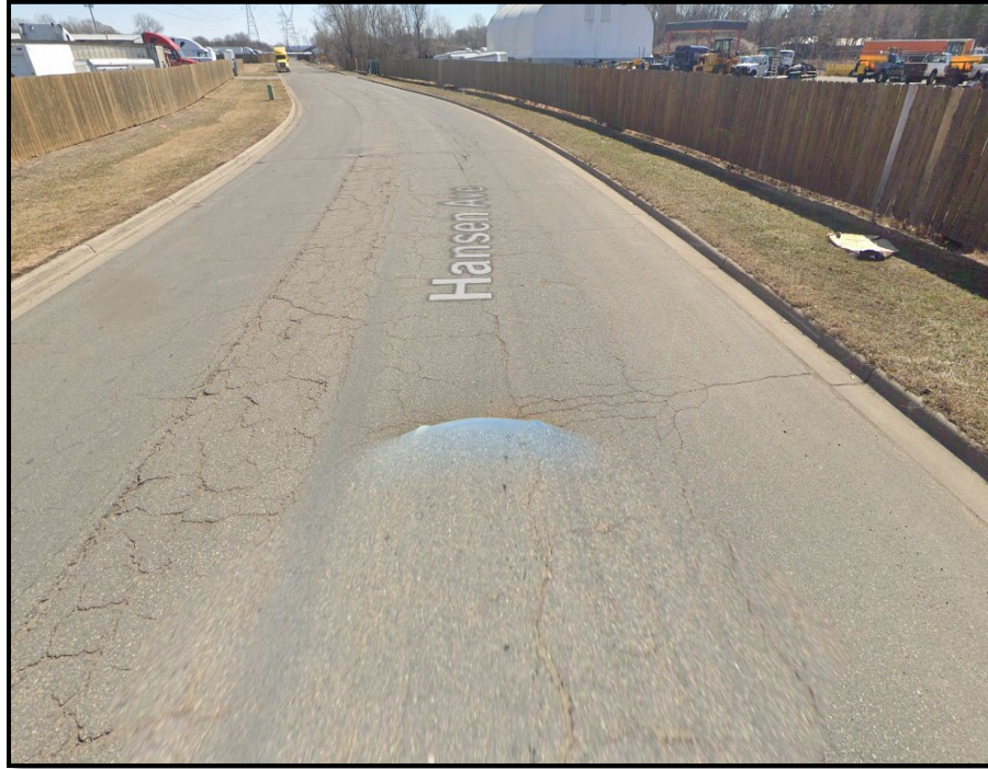
Hansen Avenue Before Construction
