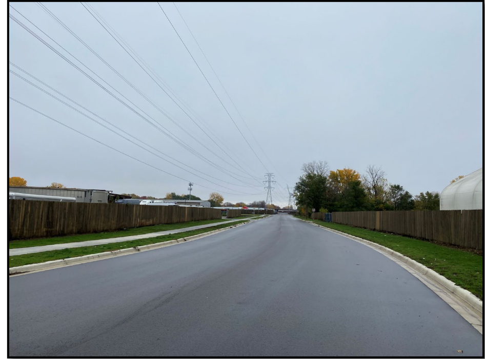
Hansen Avenue After Reconstruction
