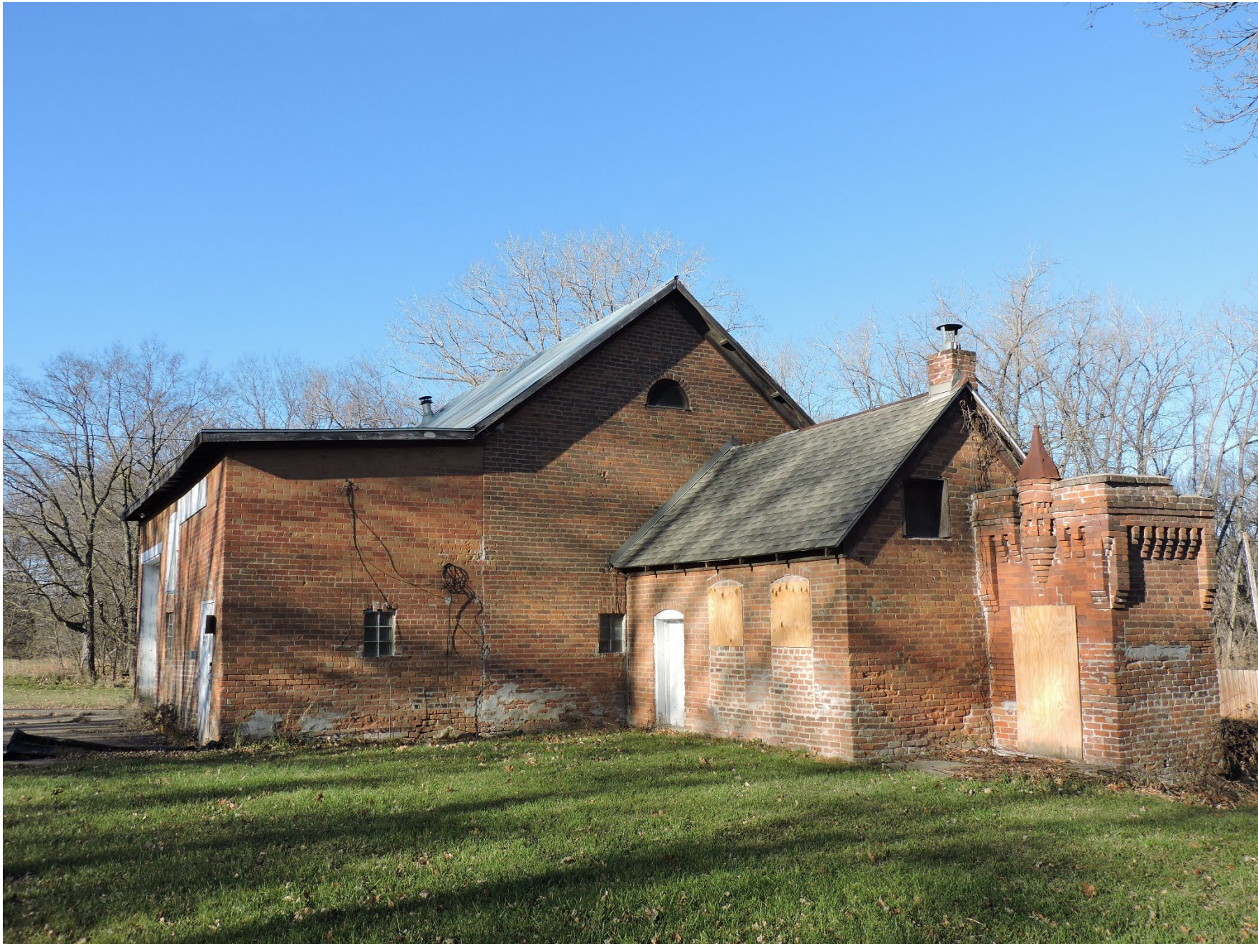
MN_Scott County_Herman Schroeder House and Livery_0023 View of Livery (contributing), east elevation with outhouse at right, looking west-northwest
