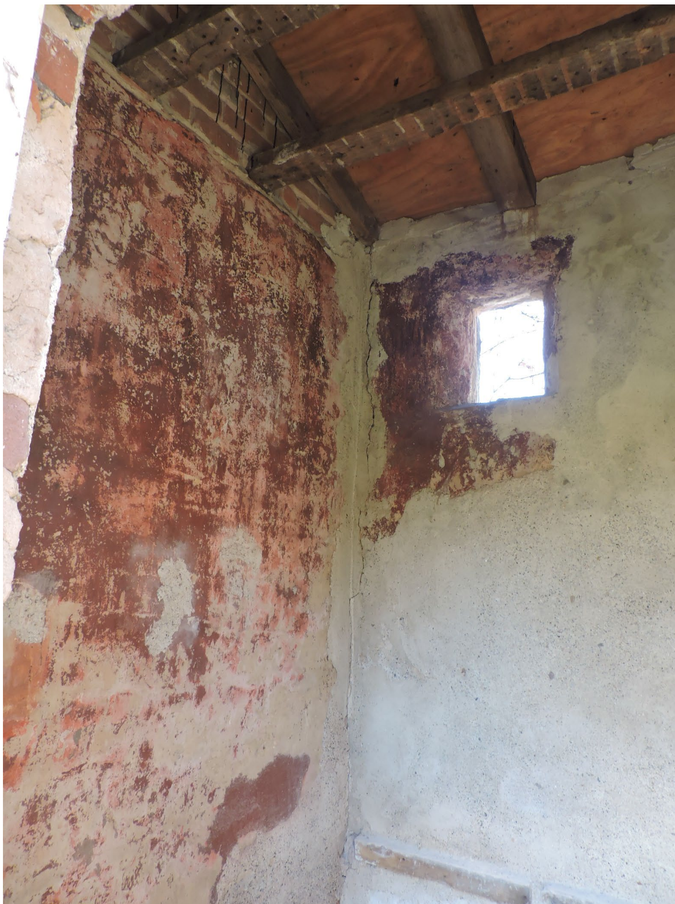
MN_Scott County_Herman Schroeder House and Livery_0028 View of Livery (contributing), outhouse, looking northwest
