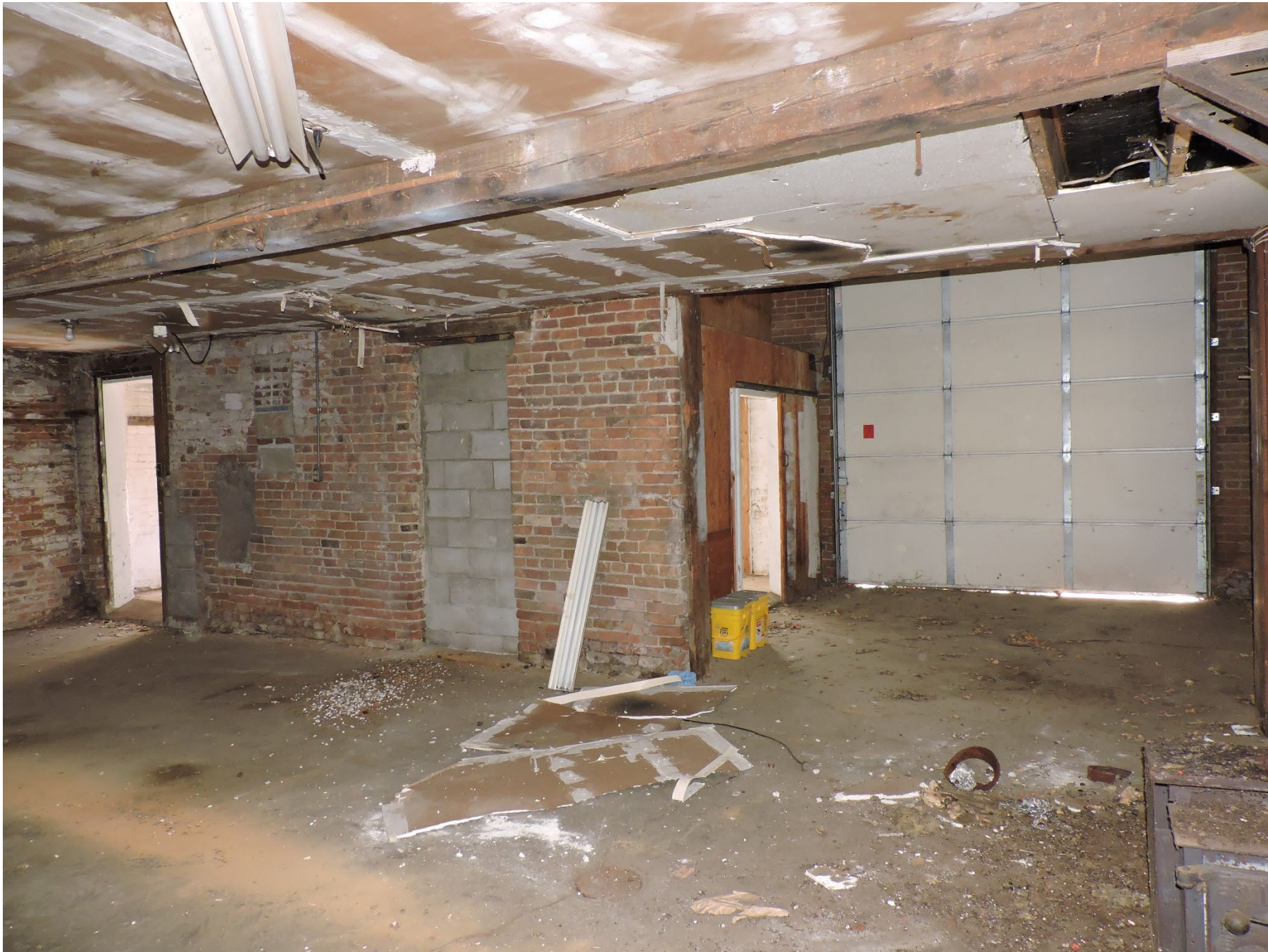
MN_Scott County_Herman Schroeder House and Livery_0025 View of Livery (contributing), north and southwest rooms, looking southeast
