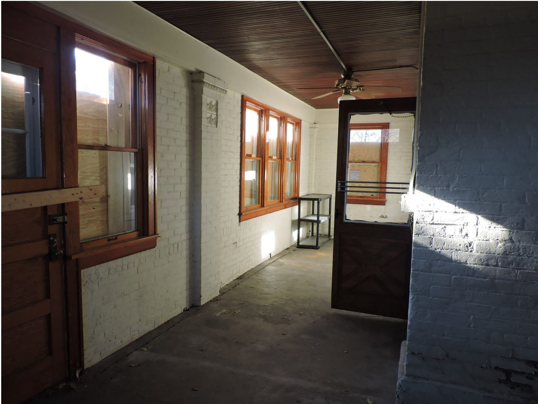
MN_Scott County_Herman Schroeder House and Livery_0013 View of Herman Schroeder House (contributing), first floor porch, looking west-southwest
