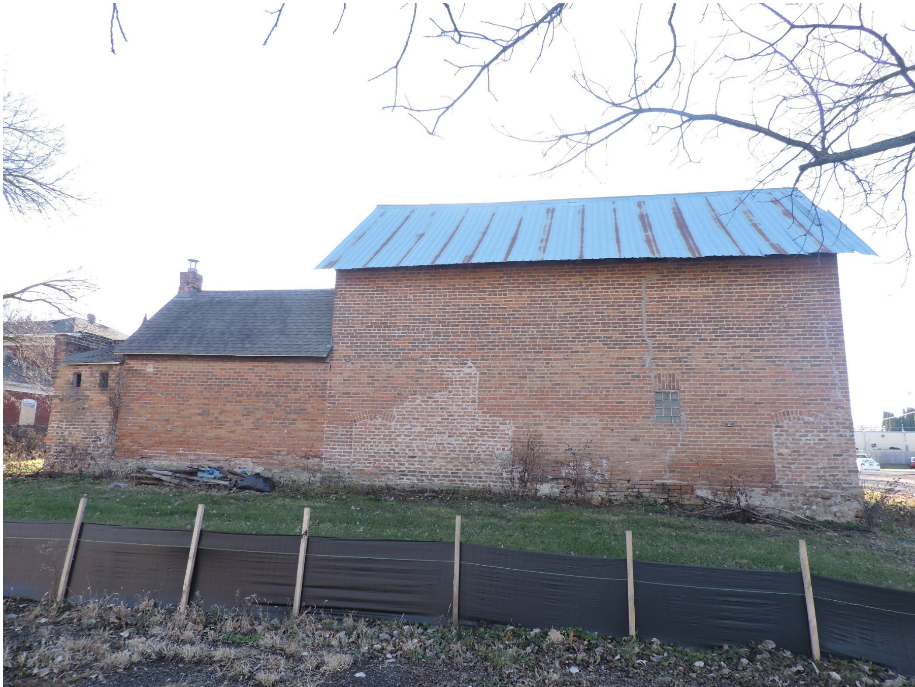
MN_Scott County_Herman Schroeder House and Livery_0021 View of Livery (contributing), north elevation, looking south
