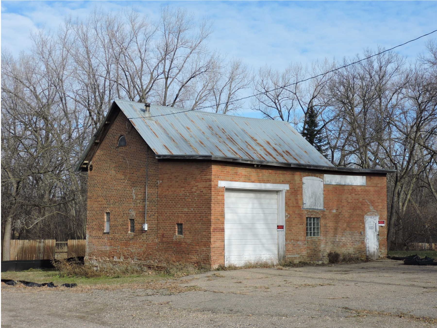
MN_Scott County_Herman Schroeder House and Livery_0019 View of Livery (contributing), west and north elevations, looking northeast
