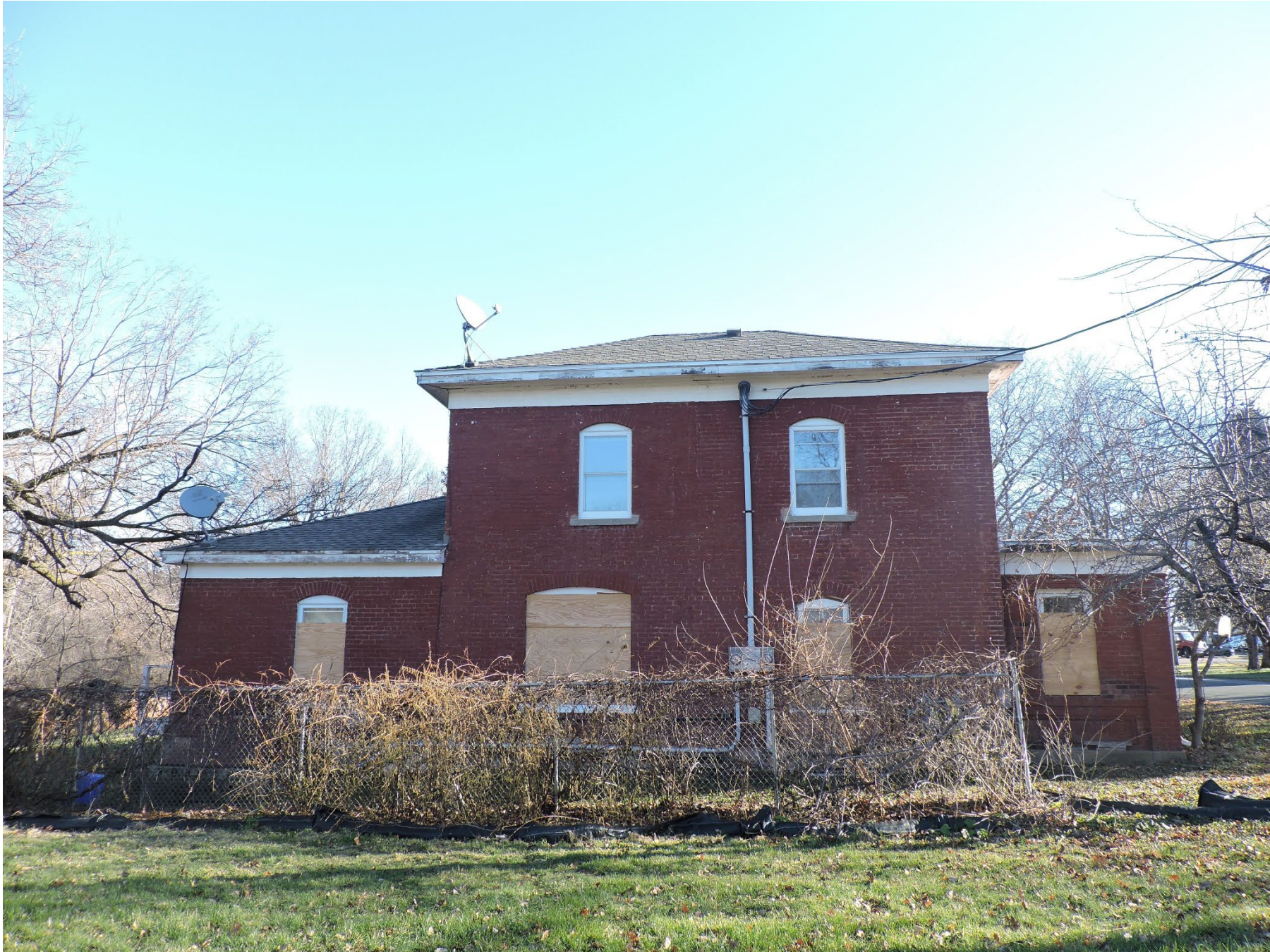
MN_Scott County_Herman Schroeder House and Livery_0007 View of Herman Schroeder House (contributing), west elevation, looking east
