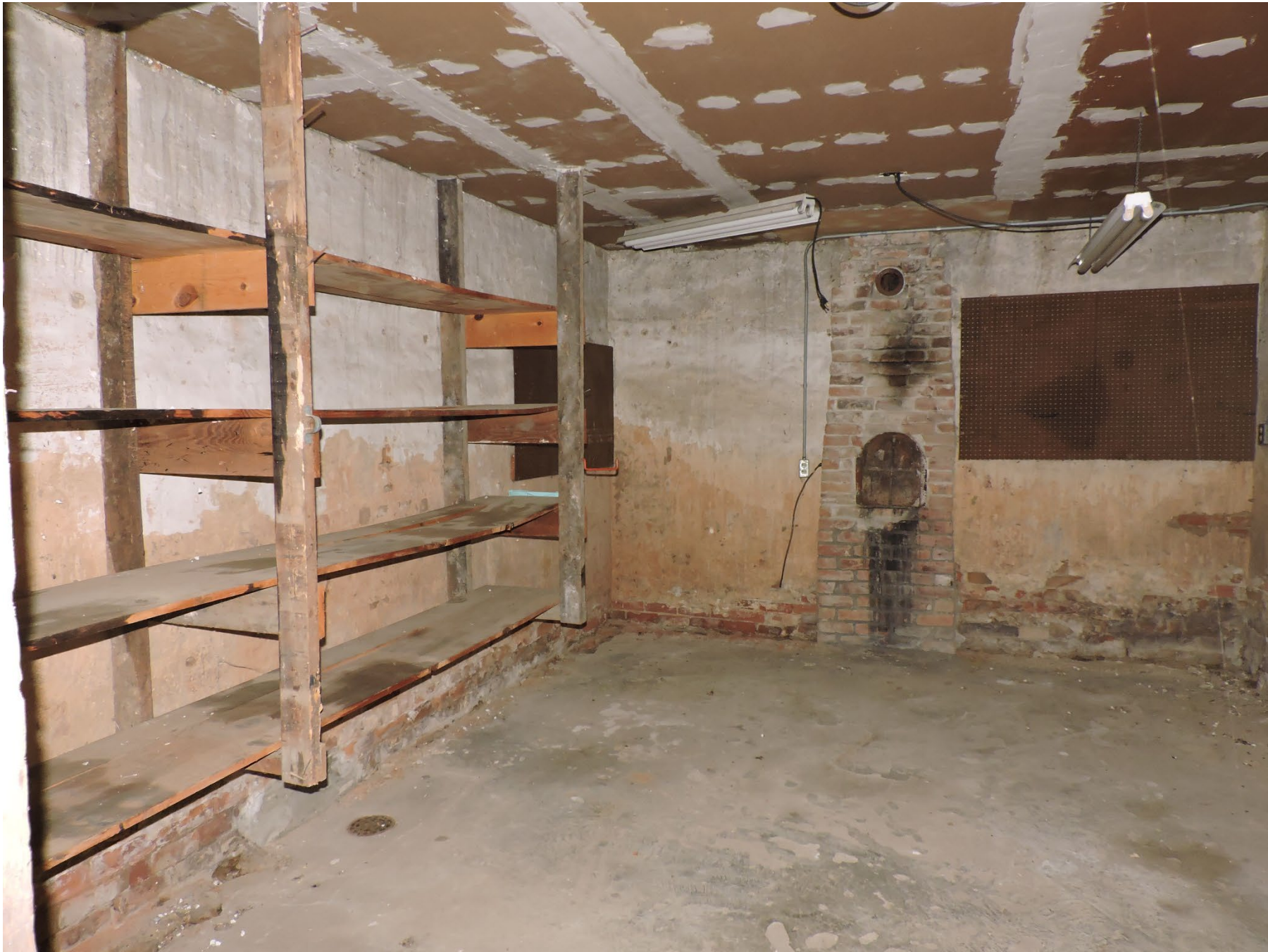
MN_Scott County_Herman Schroeder House and Livery_0027 View of Livery (contributing), side-gabled addition, looking east-northeast
