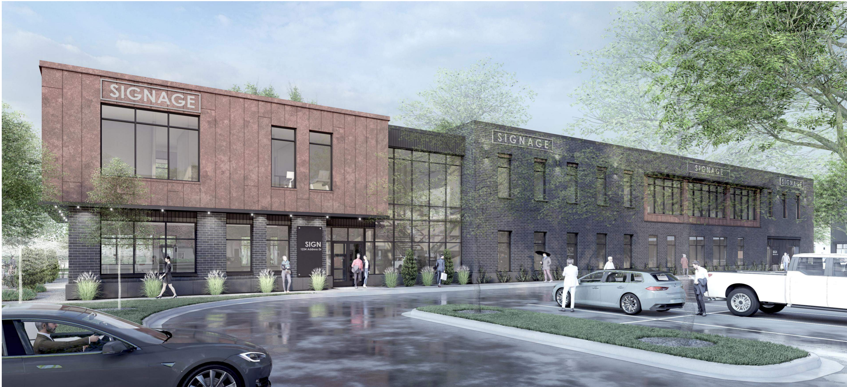
Image 3 - view from south (parking lot)
