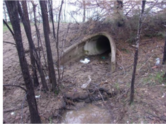
30" RCP from the east.
