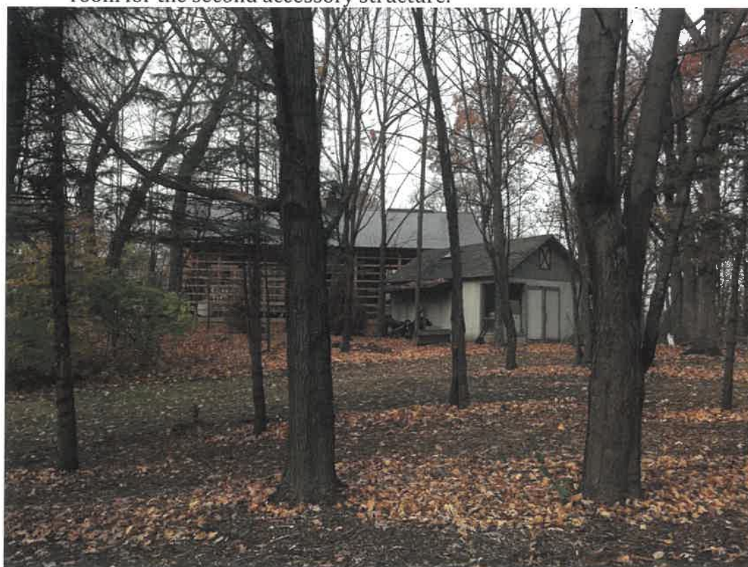
Picture 6: October 30, 2018 – Same area as picture 2 showing the incomplete second accessory structure.
