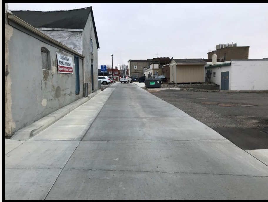
Shakopee Avenue – After Construction
