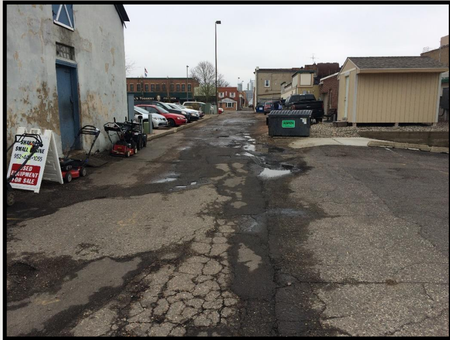
Shakopee Avenue – Before Construction
