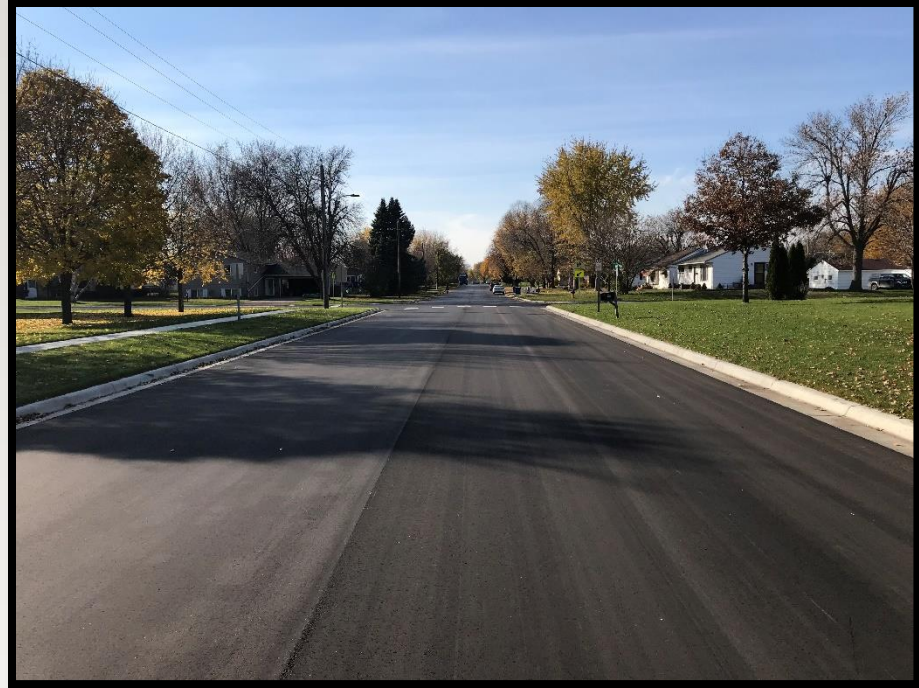
Shakopee Avenue – After Construction
