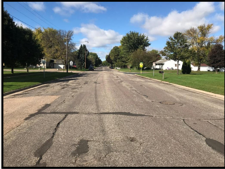
Shakopee Avenue – Before Construction
