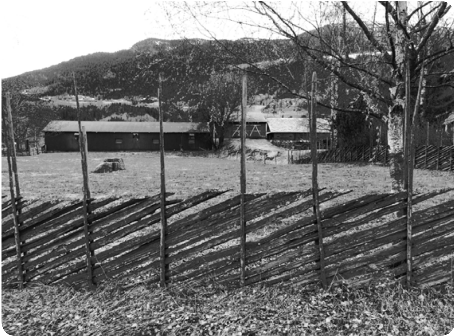
The roundpole fence or “Skigard,” is typical of the Norwegian countryside and traditionally made from unbarked and unsplit young spruce and juniper trees.
