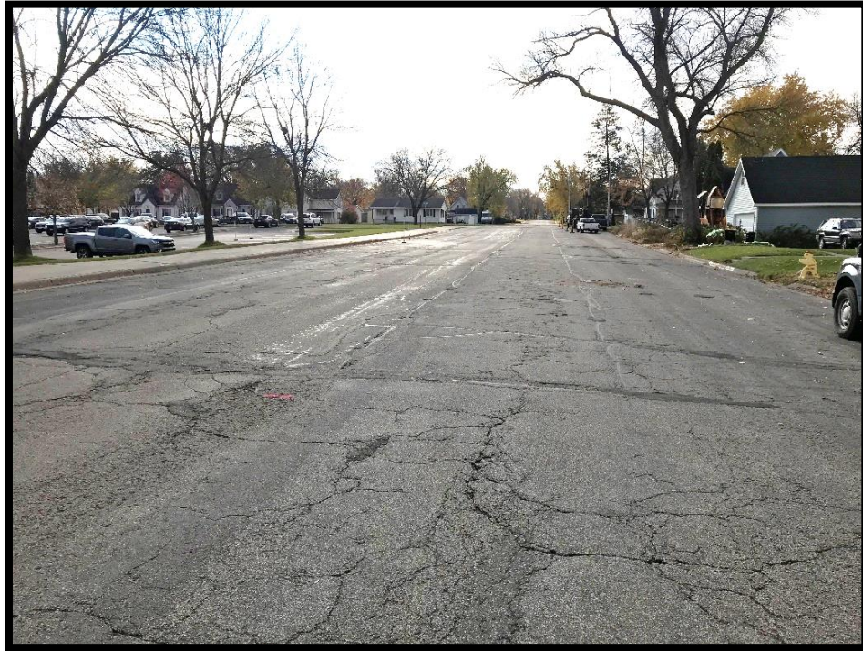
Scott Street Before Construction
