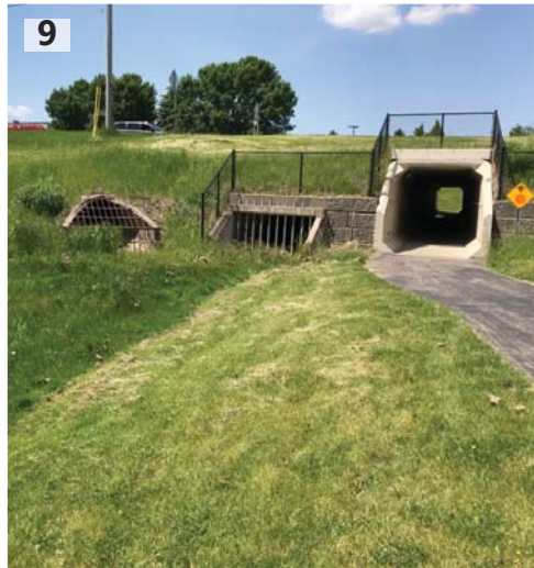
9 WEEDY AND UNWELCOMING INFRASTRUCTURE DEFINE TUNNEL CROSSINGS AND CULVERTS.
