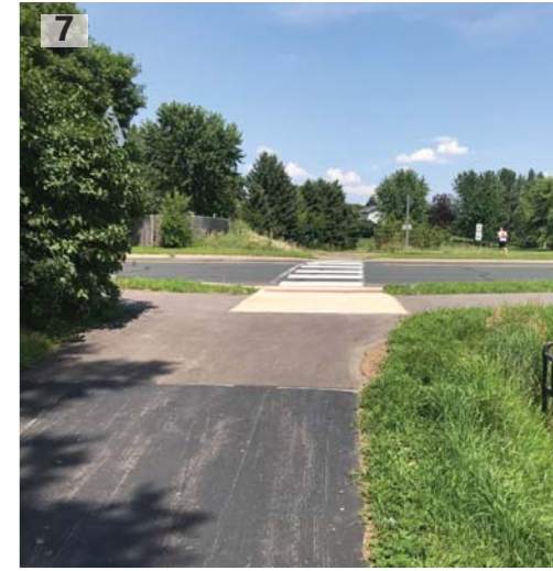
7 THIS VIERLING DRIVE CROSSING IS BLIND AND CHALLENGING TO NAVIGATE AS THE TRAIL IS OFFSET ON EITHER SIDE OF THE STREET, REQUIRING TRAIL USERS TO USE THE CITY SIDEWALK FOR A SMALL RUN.
