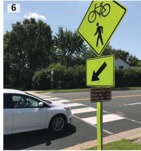
6 TRAIL CROSSING SIGN AND ROAD STRIPING ALERTS DRIVERS OF TRAIL USERS. AT A GREATER SCALE, THE AT-GRADE TRAIL CROSSING MARKINGS ARE MINIMAL AND COULD BE IMPROVED UPON FOR SAFETY.
