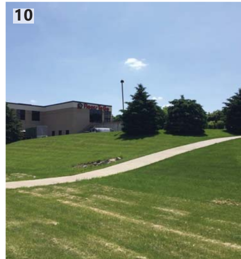
10 AN EXAMPLE OF A NEWER PATH THAT CONNECTS TRAIL USERS TO AN ADJACENT COMMERCIAL NODE.
