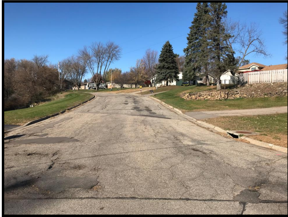
Park Ridge Drive Before Construction
