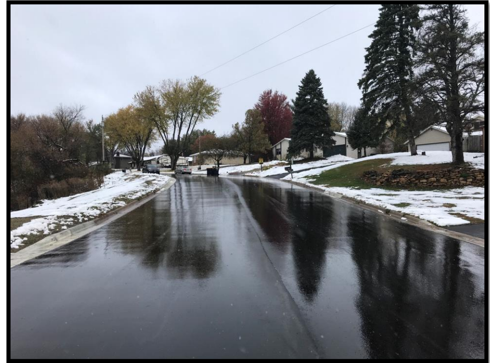
Park Ridge Drive After Reconstruction
