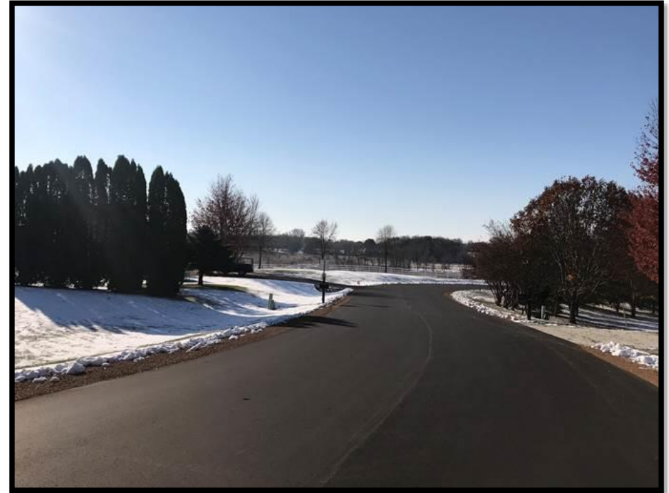
Vista Ridge Drive After Reconstruction
