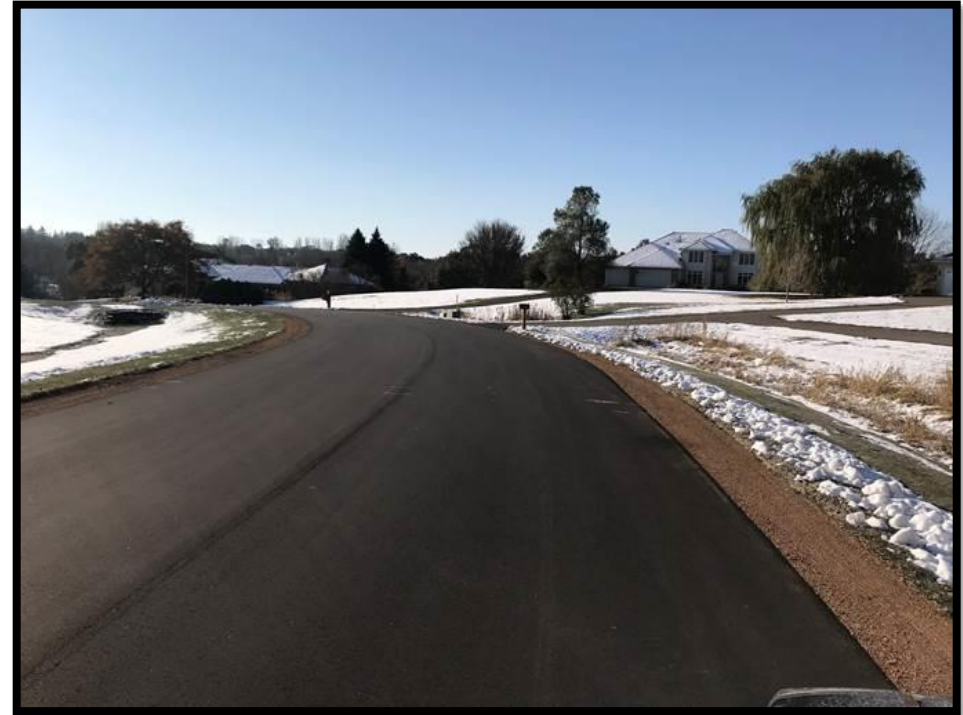
Dominion Hills After Reconstruction
