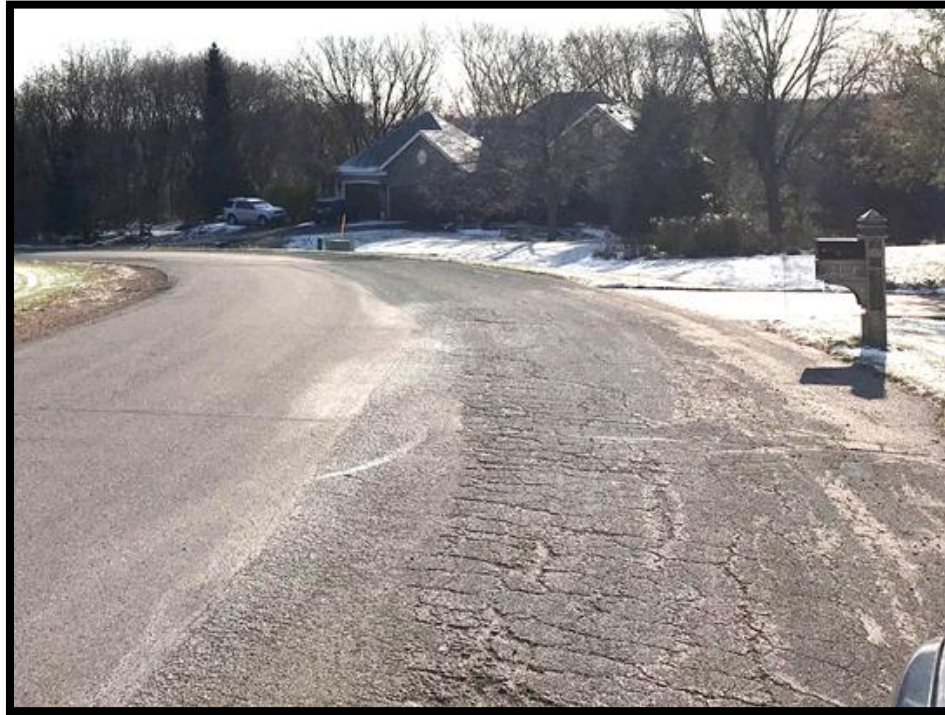
Dominion Hills Before Construction
