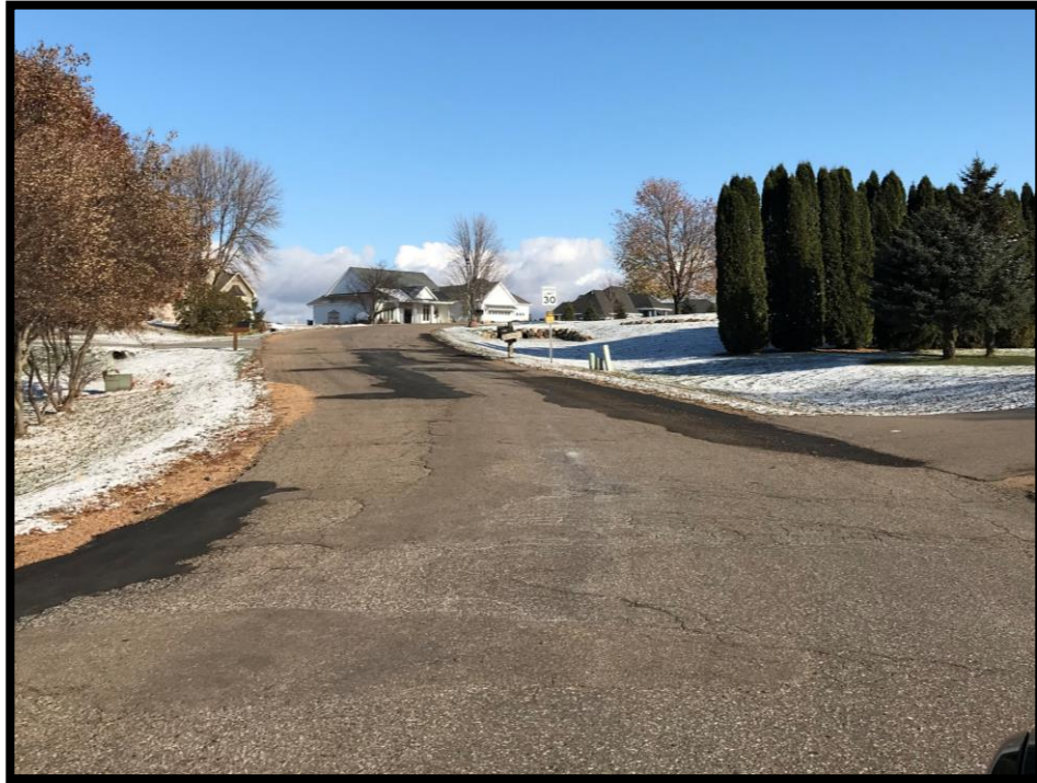
Vista Ridge Drive Before Construction
