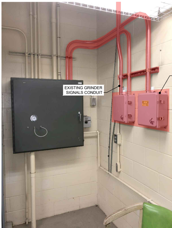
4 E104 L16 OMNI MONITORING SYSTEM REMOVAL
