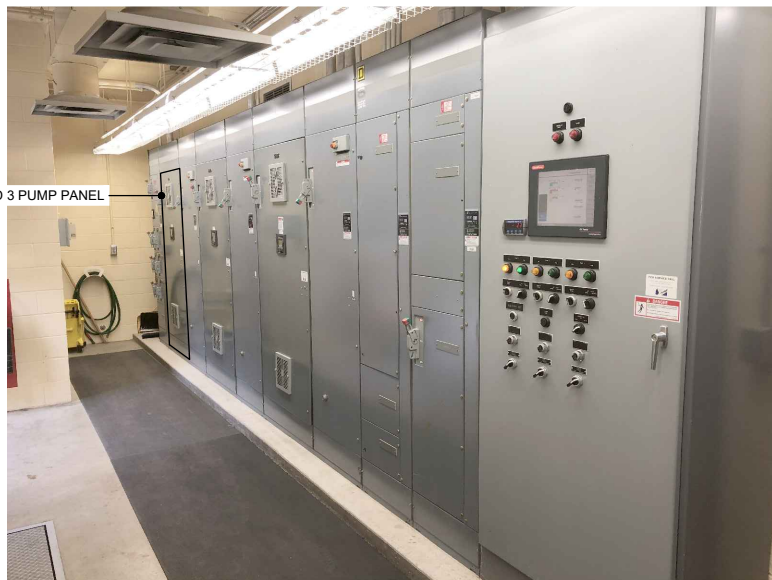
5 E104 L16 MCC AND CONTROL PANEL LAYOUT
