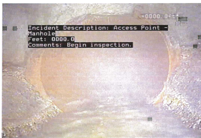
AMH - Access Point - Manhole @ 0.0 ft. Begin inspection.
