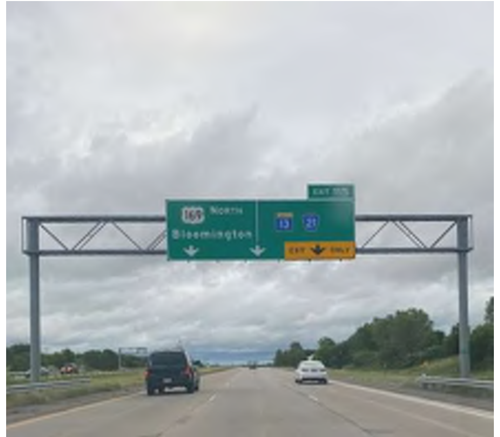
Figure 11 – Sign Bridge on Eastbound TH 169 – 2
