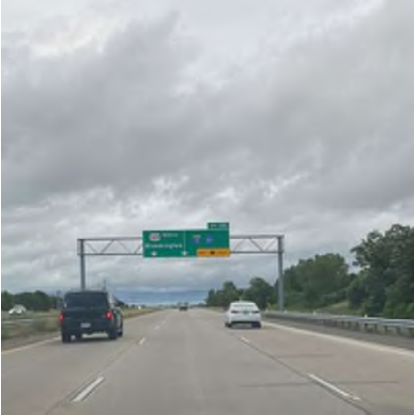
Figure 10 – Sign Bridge on Eastbound TH 169 – 1
