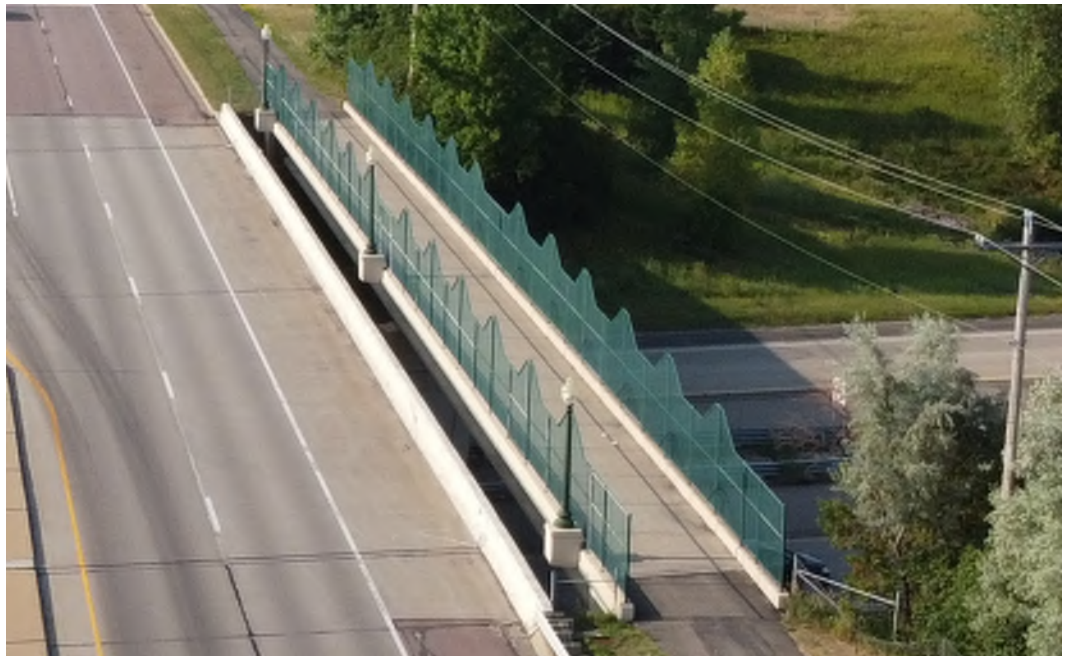
Figure 13 – Marschall Road Pedestrian Bridge over TH 169 – 2
