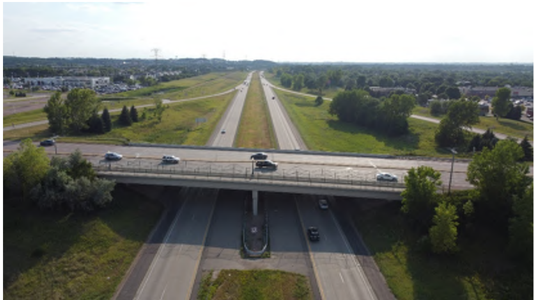
Figure 12 – Marschall Road Pedestrian Bridge over TH 169 – 1
