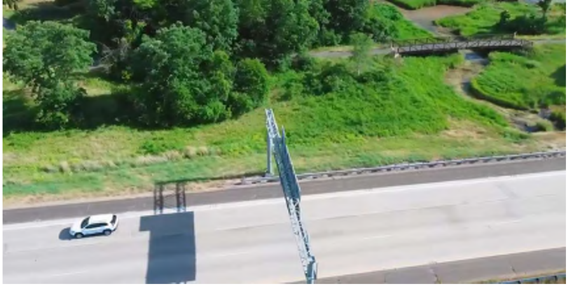
Figure 2 – Existing Conditions Looking South
