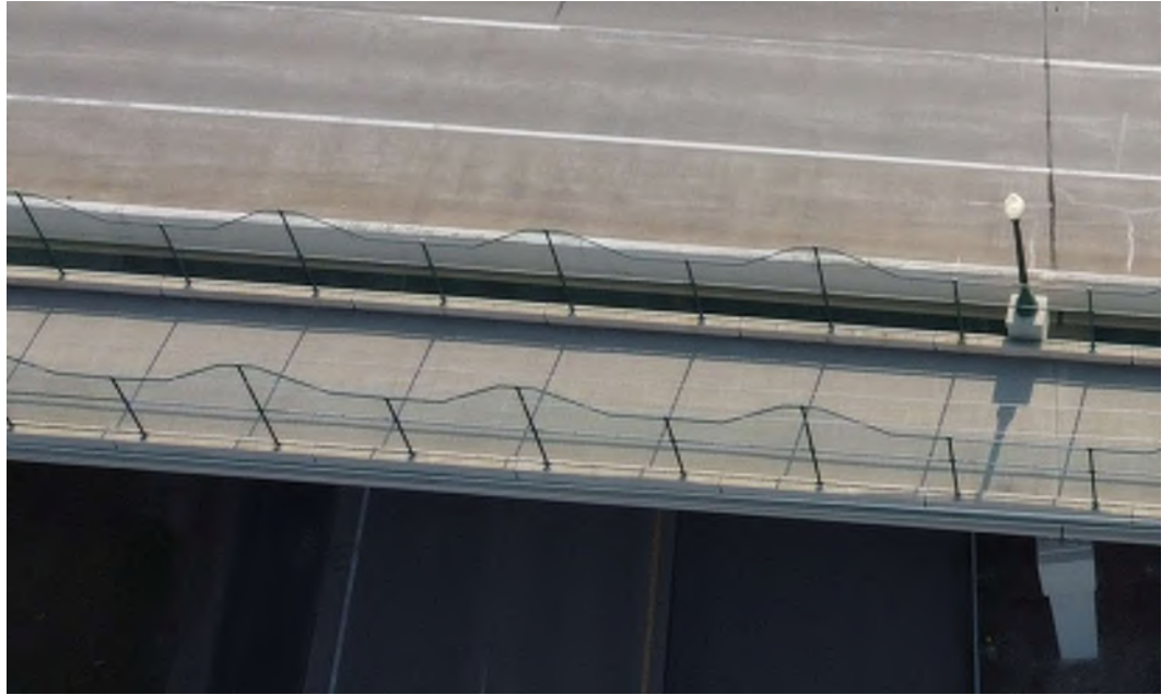
Figure 14 – Marschall Road Pedestrian Bridge over TH 169 – 3
