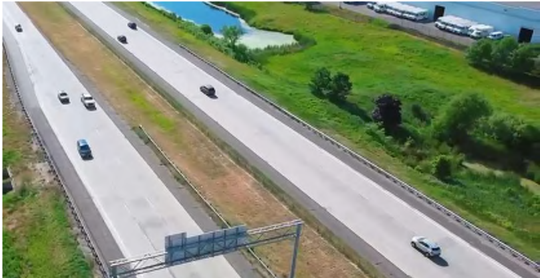
Figure 3 – Existing Conditions Looking North
