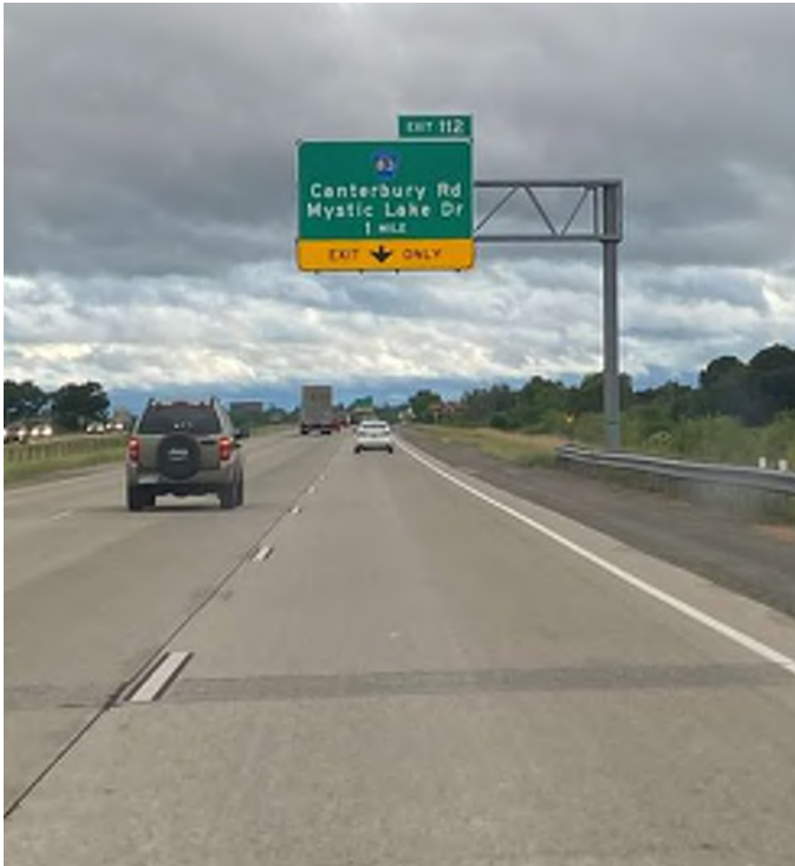
Figure 7 – Sign Bridge on Westbound TH 169 – 1
