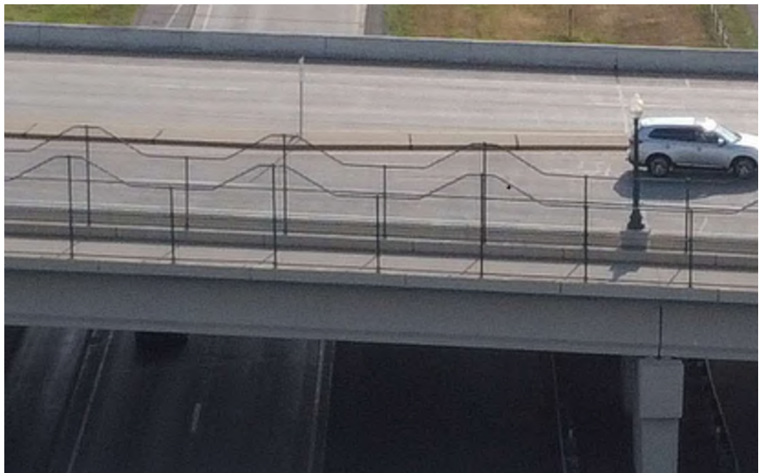
Figure 15 – Marschall Road Pedestrian Bridge over TH 169 – 4
